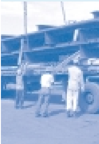
Bridge bed panels being loaded aboard trucks at Palua Port, Venezuela.
